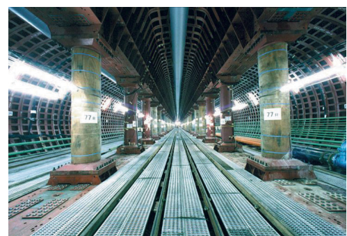
▲ Construction in the lidabashi station work section in a loop on subway line No. 12 (cross section: 17.44 m wide and 8.846 m high)
