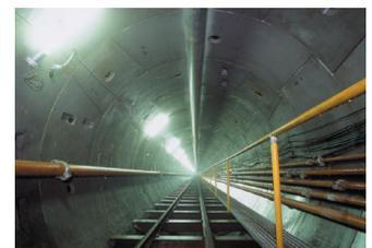
▲ Midorigaoka Rainwater Trunk Line of Sagami City Public Drain Construction Work (Lining Outer Diameter: 3,120 mm)
