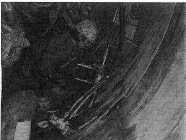
Fig. 15. Circumferential tensioning.
