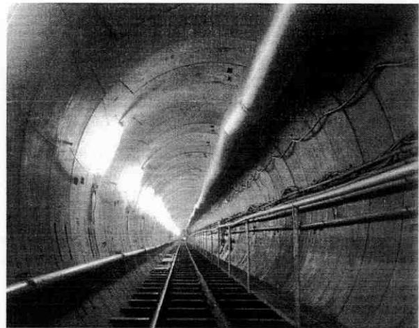
Fig. 17. Overall view of inside of tunnel.
