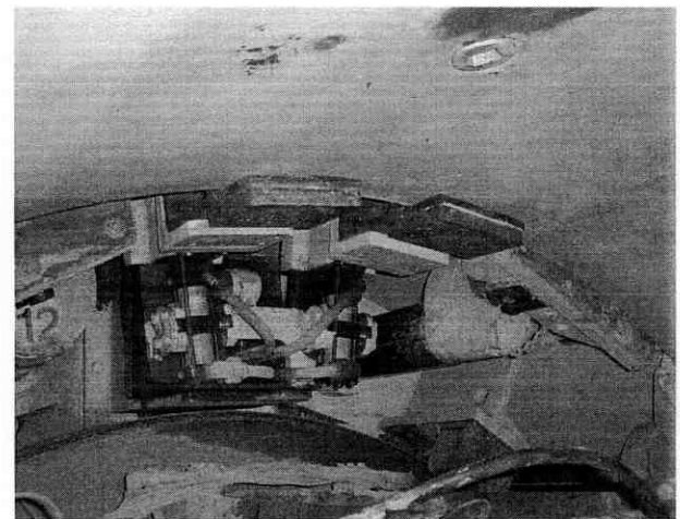
Fig. 11. Temporary support jack.
