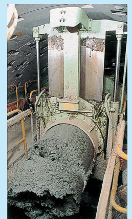
Excavated soil discharged from the screw conveyor
