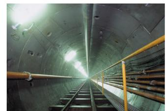
▲ Midorigaoka Rainwater Trunk Line of Sagamiara City Public Drain Construction Work (Lining Outer Diameter: 3,120 mm)
