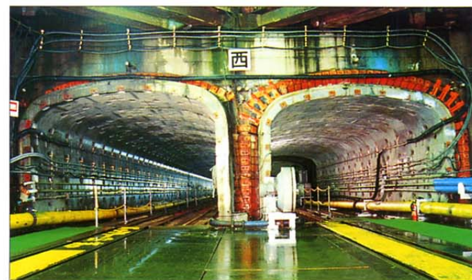
一次覆工(往路・復路) Primary lining of outgoing and return tunnel (outgoing and return tunnels)
