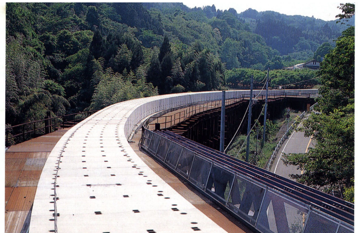
Hokuriku Shinkansen Akima Tunnel East Project
